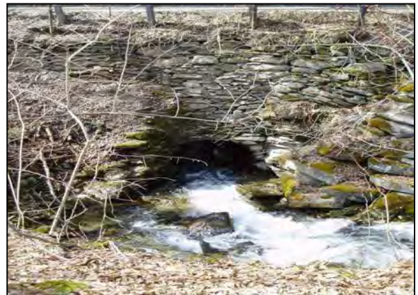
Figure 12: Stone arch bridge on Woodcock Road.
