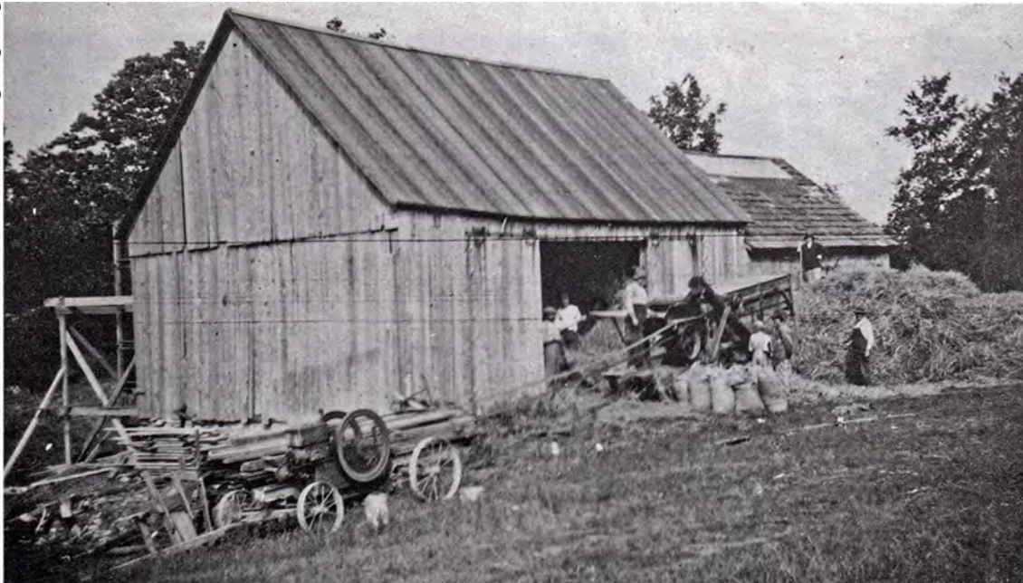
ENGLISH BARN ON THE HAGELBERG FARM. This Crow Hill Road scene shows threshing, probably oats, being done right at the barn door. The English barn was the most common 19th-century barn type on Vermont farms. It has the main entrance with double-leaf sliding doors in the central bay of the eaves facade. The thresher is being driven by a belt from the auxiliary engine on the four-wheel chassis (left).
