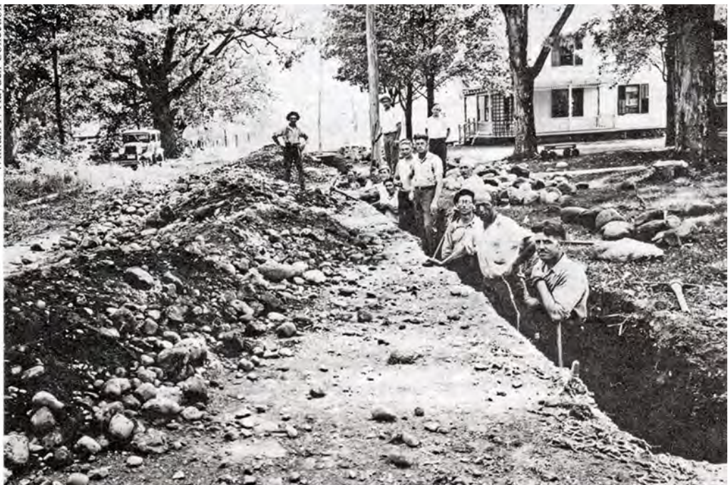
DIG THEY MUST ON WATER STREET. This crew of intrepid shovelers paused for the camera in the early 1930s while digging a trench for a new water line along the street. Probably they were glad to have such employment during the depths of the Great Depression despite the number of rounded river stones in the ground.
