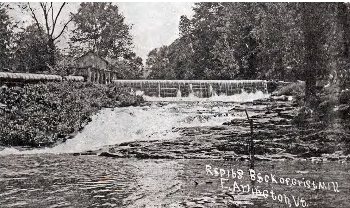
GRIST MILL DAM AND FLUME. The grist mill was powered by water delivered from the log-crib dam atop the falls through a "barrel-stave" flume seen on the left in this photograph. The wheel was mounted in the mill's stone-walled basement next to the brook. The dam was probably breached by the 1927 flood and never rebuilt.
