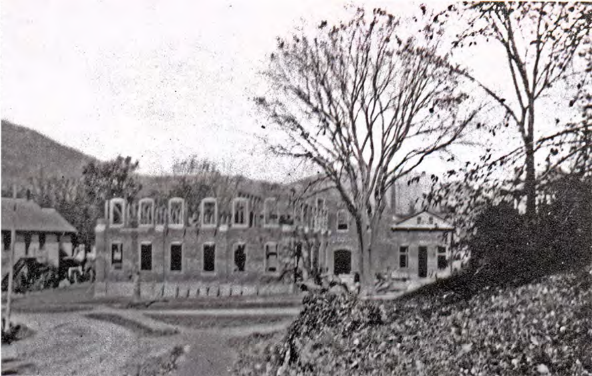
REFRIGERATOR FACTORY UNDER CONSTRUCTION. In 1910-1911 the Arlington Refrigerator Company (ARCO) erected the largest factory ever built here. This view shows the Depot Street facade at the second-story height with the wood window frames ready for the surrounding brick wall. The structure is load-bearing masonry and its design reflects an Italianate influence.
