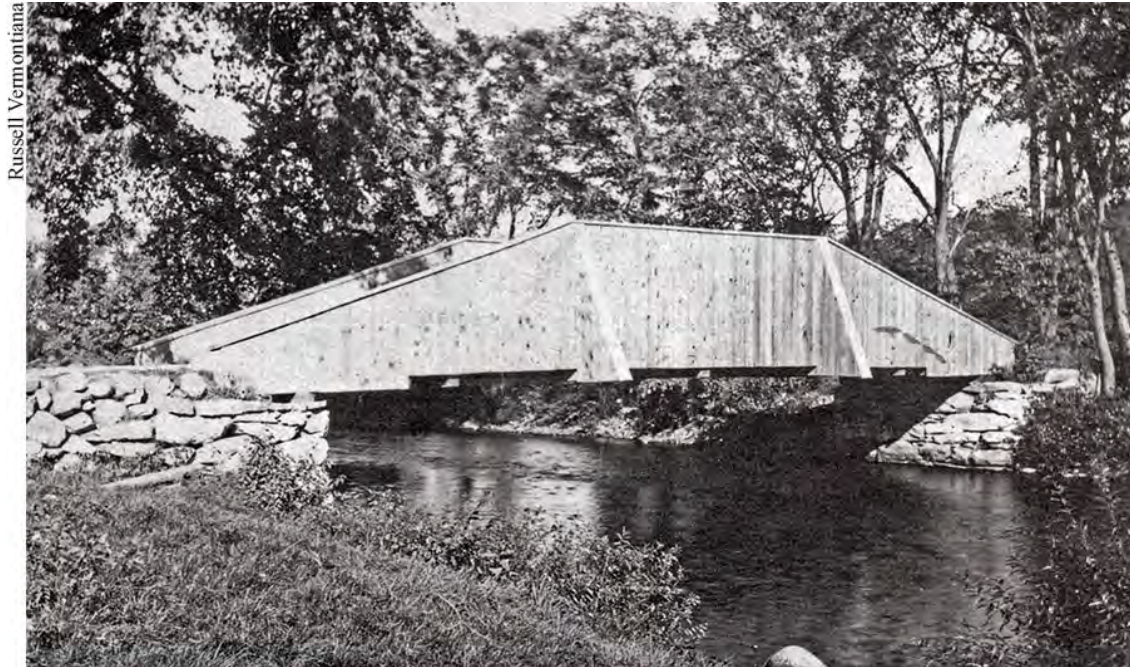
WATER STREET BRIDGE OVER THE BATTENKILL. Several road bridges of this type existed in Arlington during the latter 19th and early 20th centuries. Only the Queen post timber trusses supporting the plank deck were covered with boards for protection from the elements. (The same type of truss was also used for fully covered bridges.) This handsome example existed on Water Street (Route 313) over the Battenkill until it was destroyed by the flood of November, 1927.
